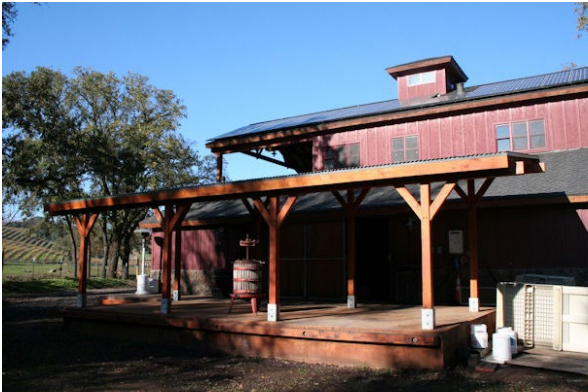
New covered crush pad, 36 solar panels on barn roof, and Geib vineyards in adjacent hills
